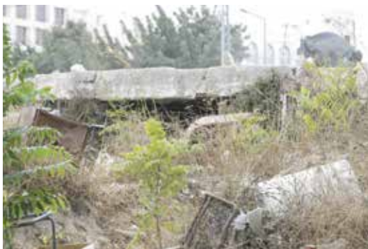
The cave entrance - zooming in from across the side road - IBN JUBAIR
