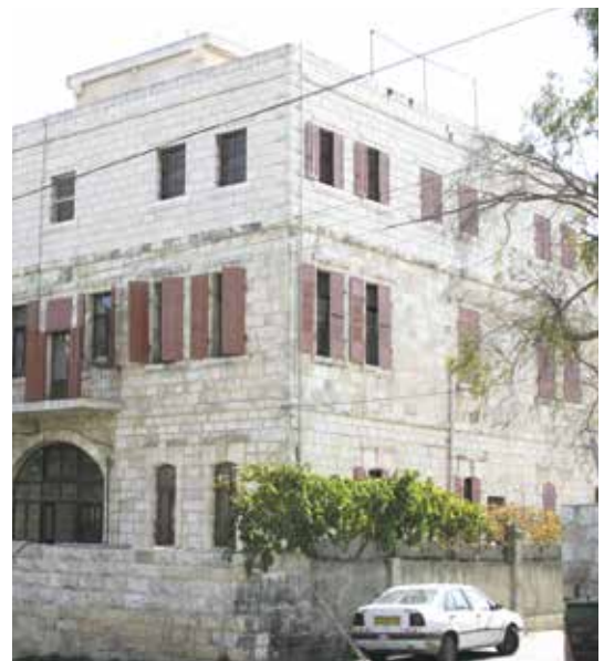
directly across this same side road - "DAR AL-AWLAD SCHOOL"
